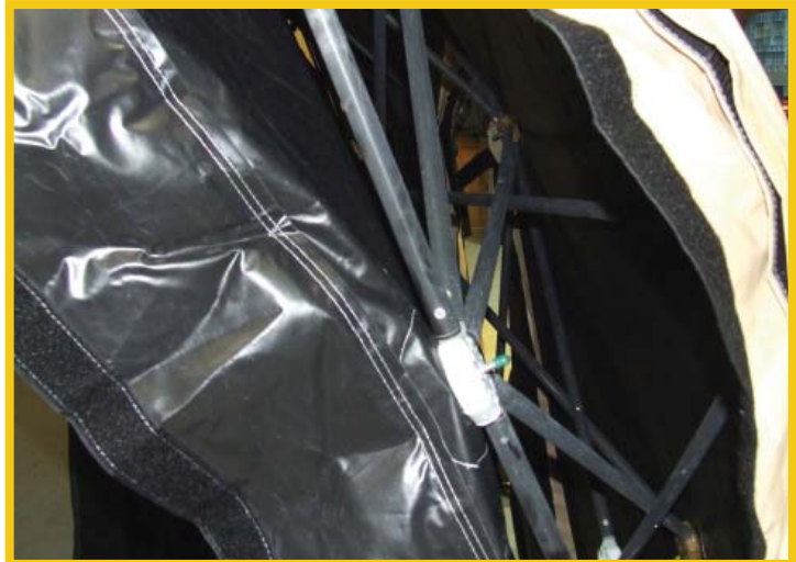
A basic component of the DRASH shelter structure, shelter struts connect at hubs to form an interlocking geodesic frame that is both durable and easy to set up.
