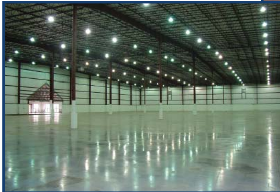
Inside the DHS Systems' 130,000 square foot facility.
