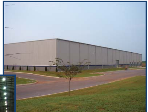
An external view of DHS Systems' Huntsville manufacturing facility.
